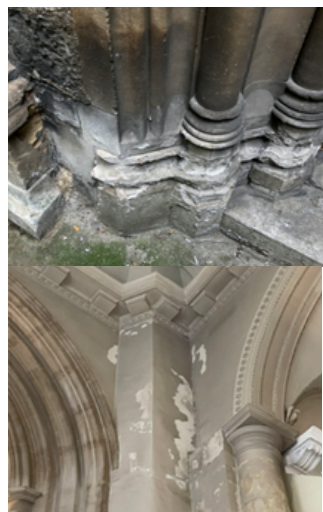
Images from the Condition Survey
